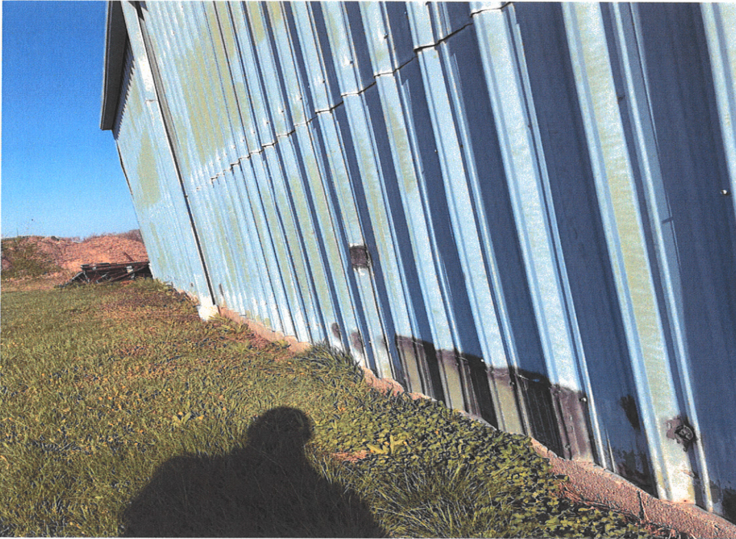
Siding repairs, typical of several areas.
