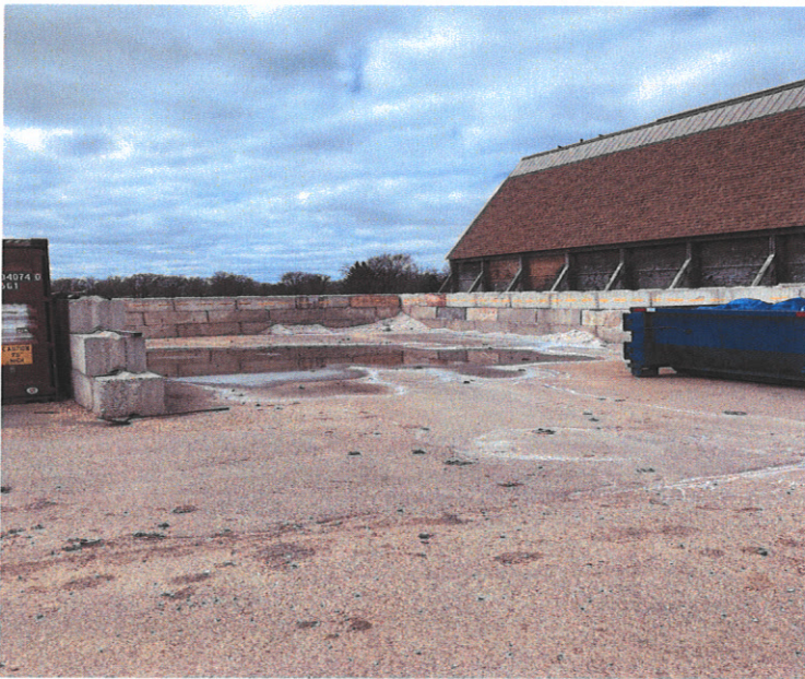
Existing outside salt storage
